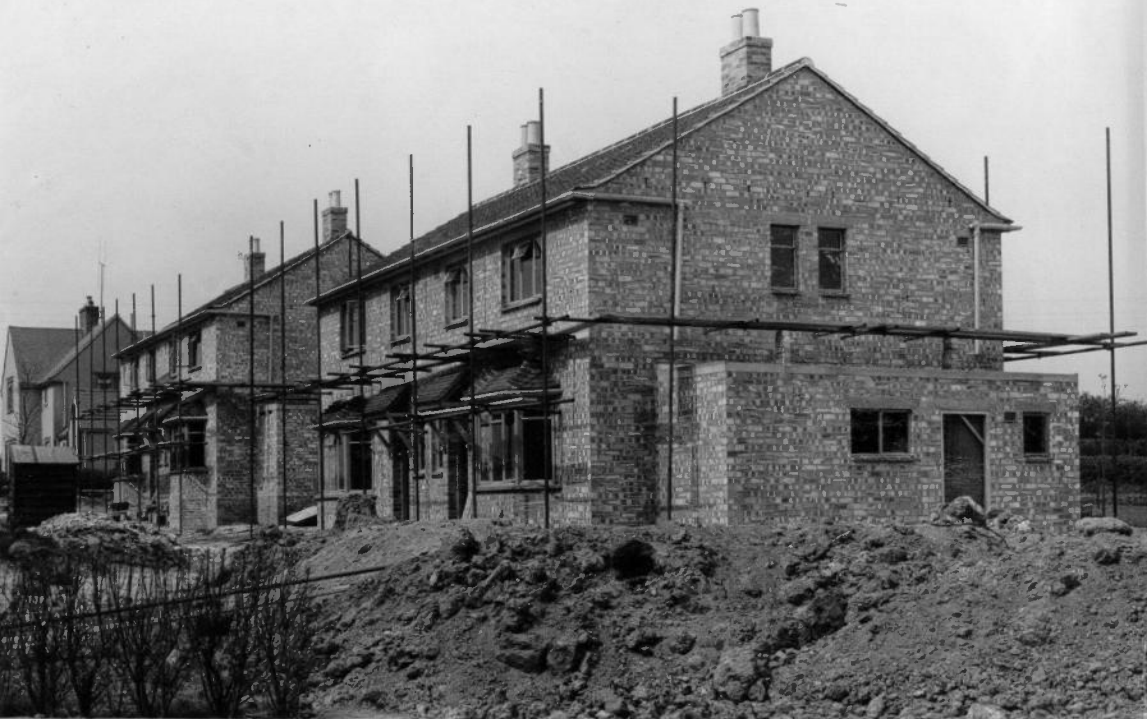
Construction of 4 New Houses at Caldecott Pumping Station - April 1954
