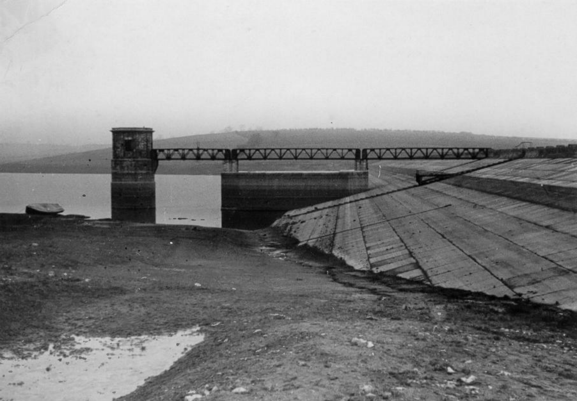
Valve Tower & Dam showing lowest level 207.8ft O.D. 10th Jan 1944
