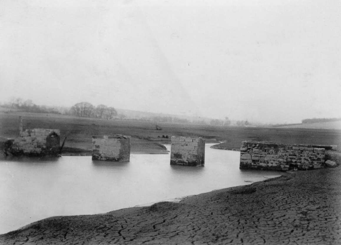
Stoke Dry bridge 20th December 1943
