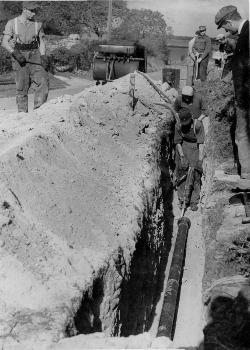
Weldon Pipe Line. Hard rock at Deene End. 1/10/46
