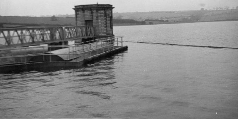
EYE BROOK RESERVOIR OVERFLOWING SUNDAY, 30TH OCTOBER 1960, 2.00 P.M. RESERVOIR LEVEL 228.14 FEET. FLOW 420 CUSECS
