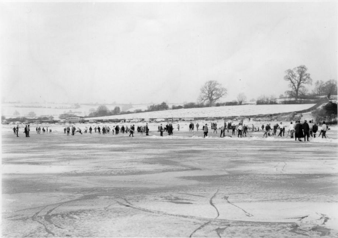
Eye Brook Reservoir completely frozen over. February, 1963.
