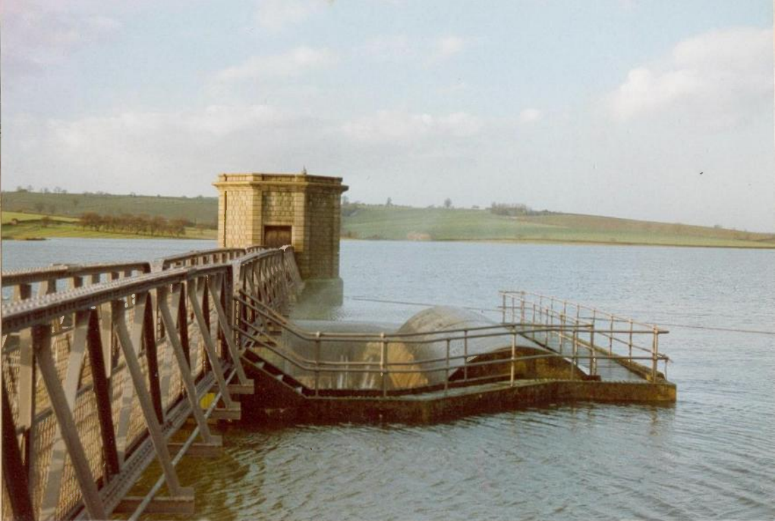
3 Siphons Worked Nos 1, 2 & 4 Peak Discharge - 512 mgd At highest level that the Reservoir reached of 228.20 ft O.D. Photograph taken on 26th January 1988
