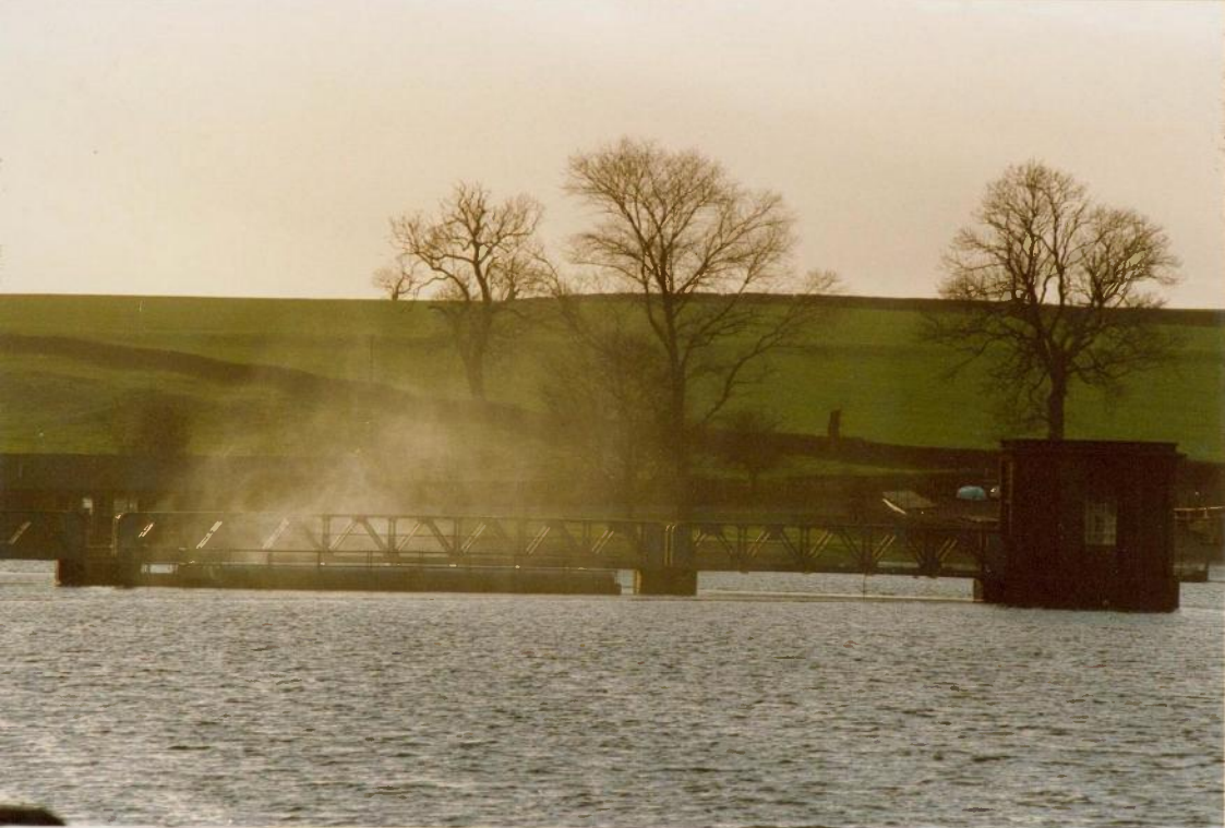
3 Siphons Worked Nos 1, 2 & 4 Peak Discharge - 512 mgd At highest level that the Reservoir reached of 228.20 ft O.D. Photograph taken on 26th January 1988
