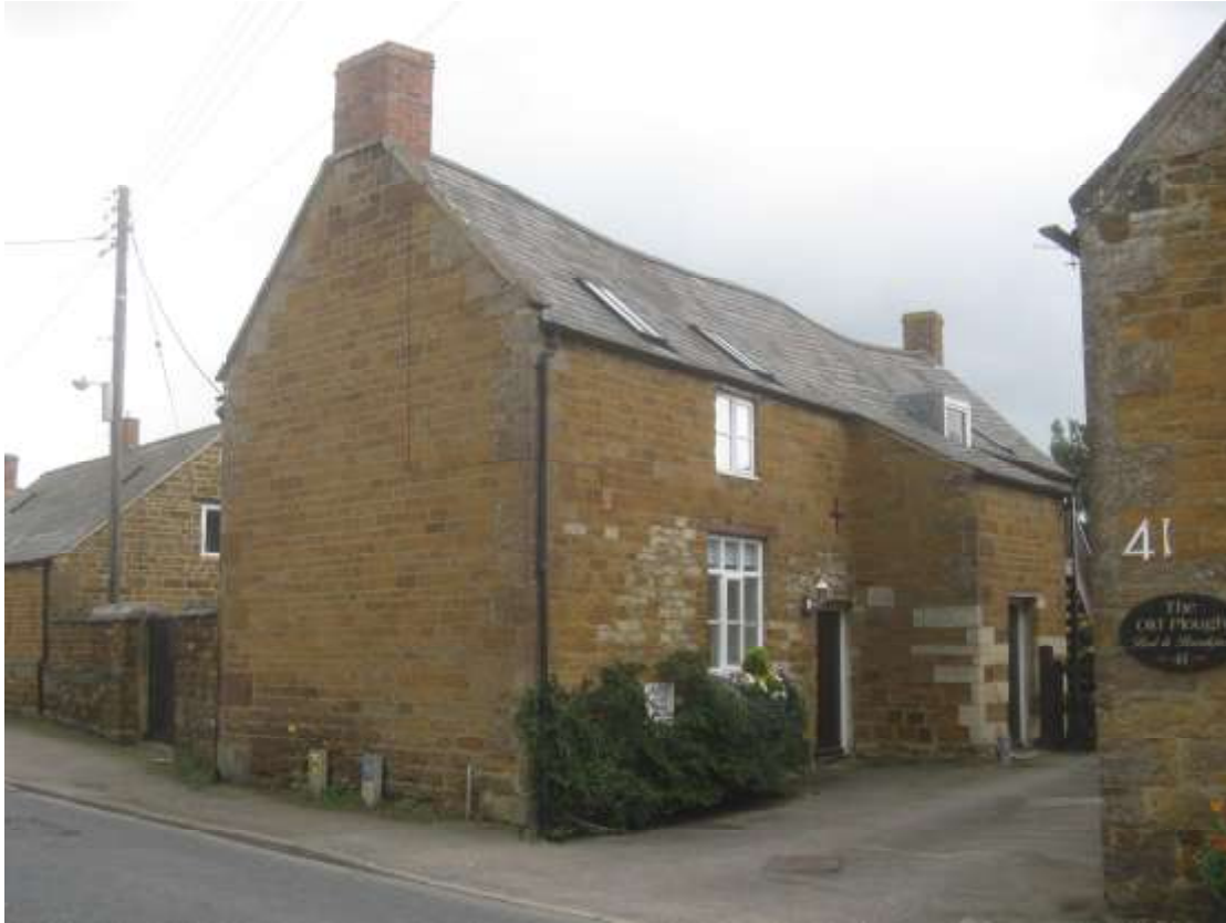
East outbuilding from north-west
