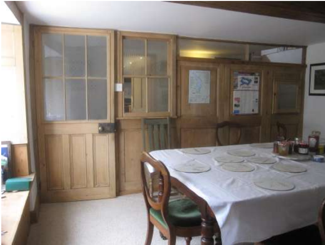
Pine partition, with doors and serving hatches; entrance passage beyond
