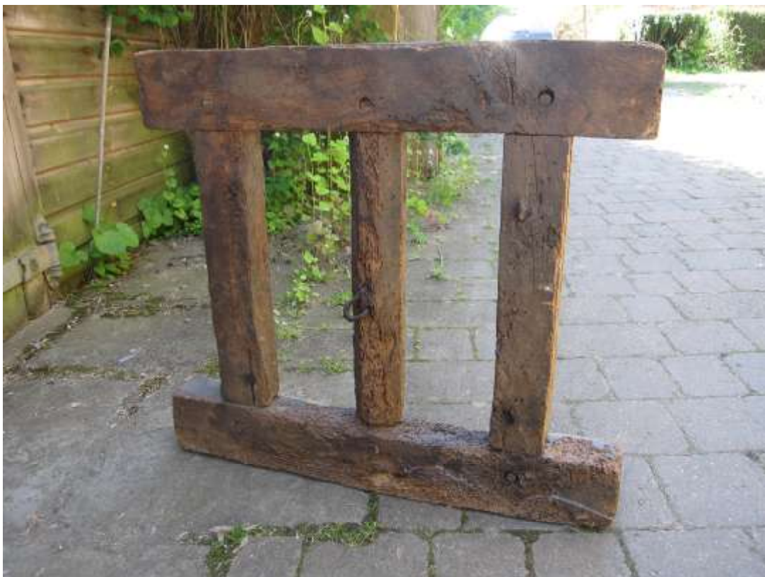
External and internal views of the C17th unglazed oak window from the parlour
