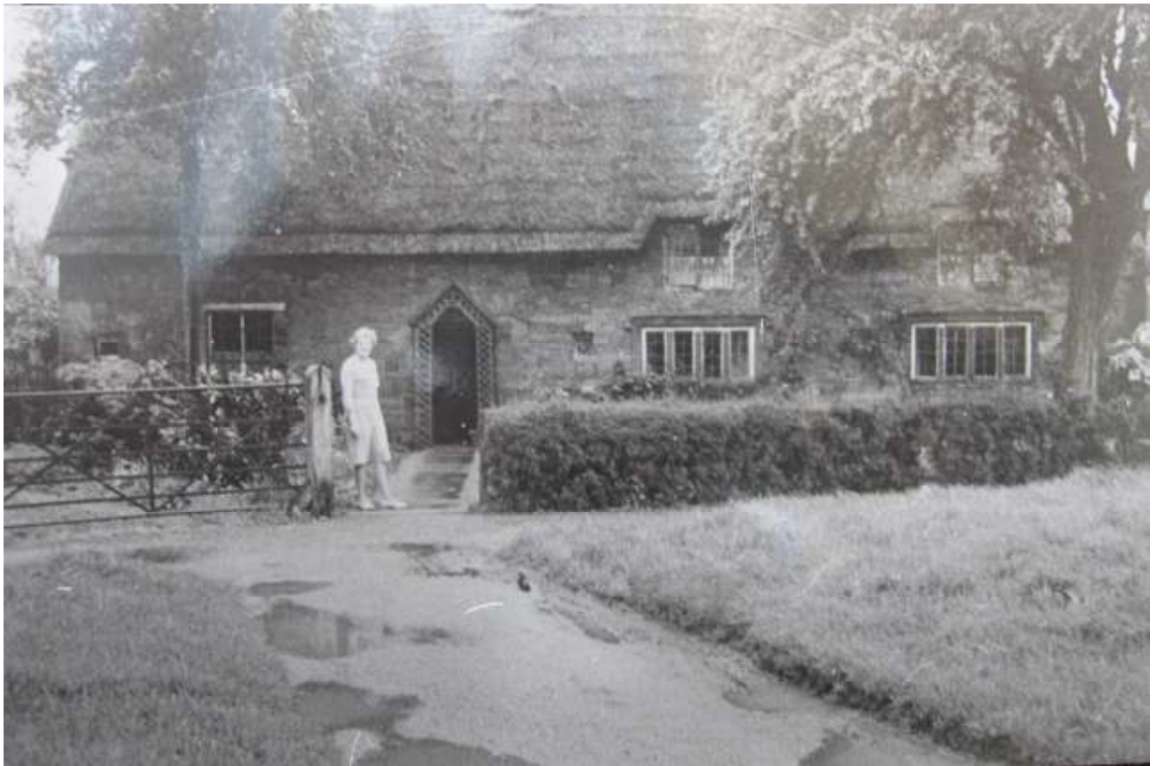
Early photograph showing roof of longstraw thatch, with eyebrow dormer windows
