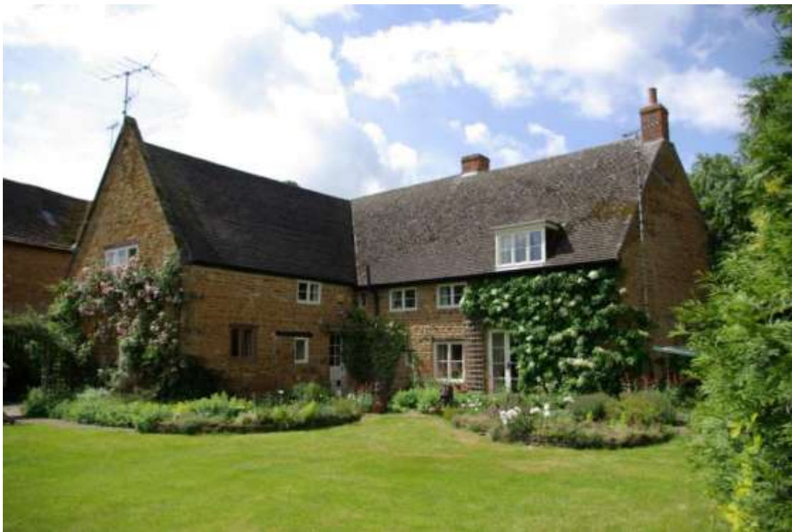
Rear view in 2009 (before addition of conservatory)
