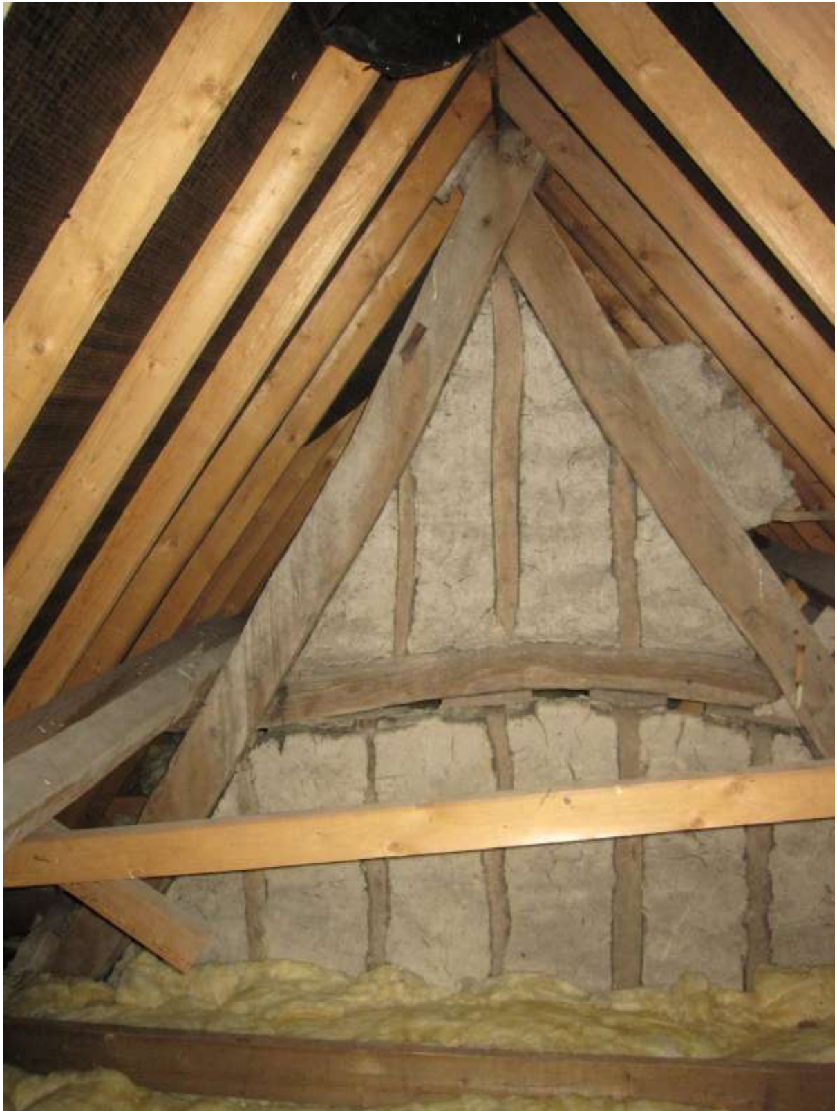
South face of truss T1 to rear wing, dated 1691-6.
