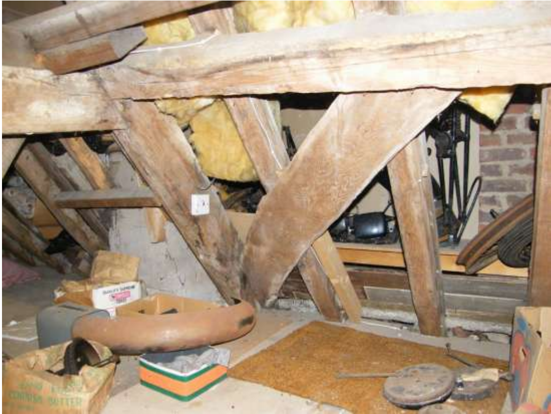
South side of Truss T3 with purlin and wind-brace
