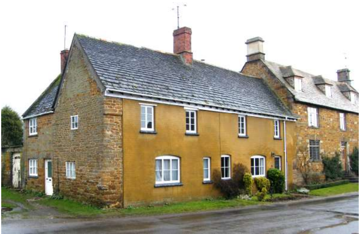
View from north-west, with No 1 to left and No 24 to right
