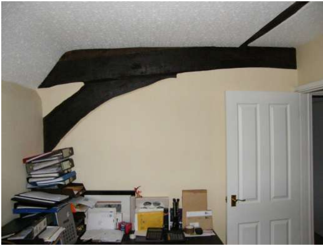
South face of Truss T3 in No 24
