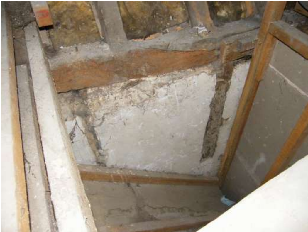
Surviving original infill panel to rear wall of No 1
