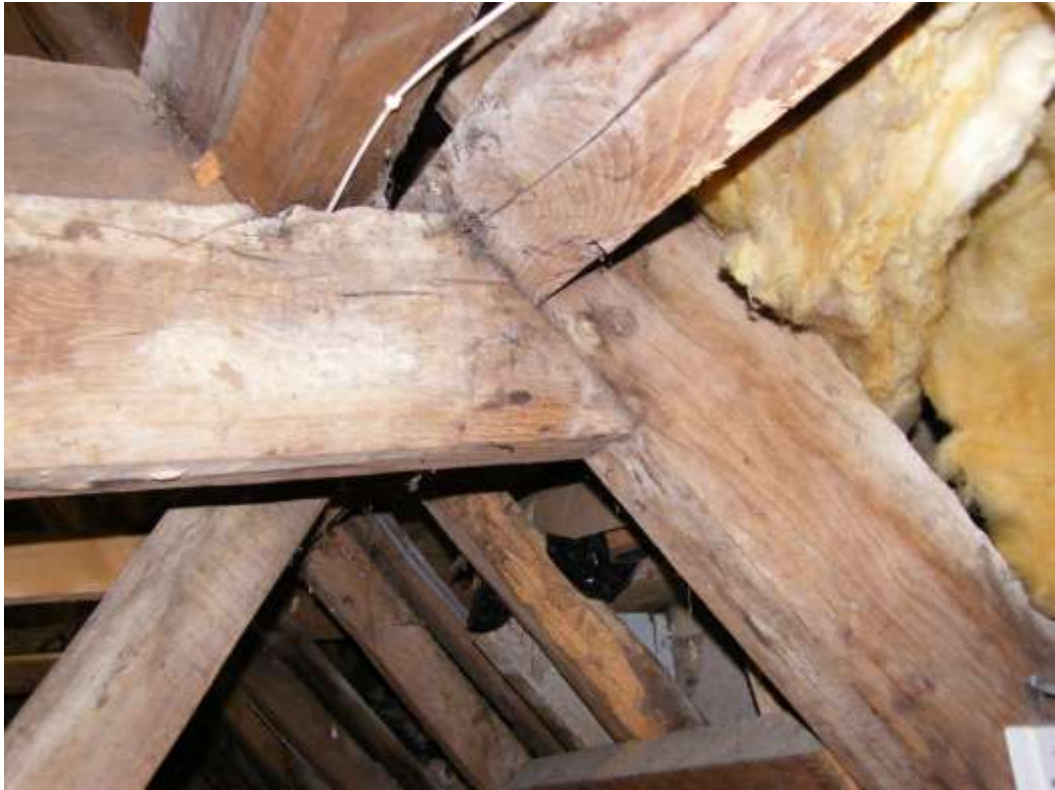
Detail as above, showing clapped purlin joint
