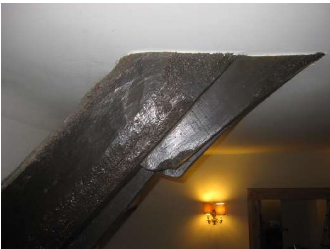
Ogee-shaped foot to arch-brace
