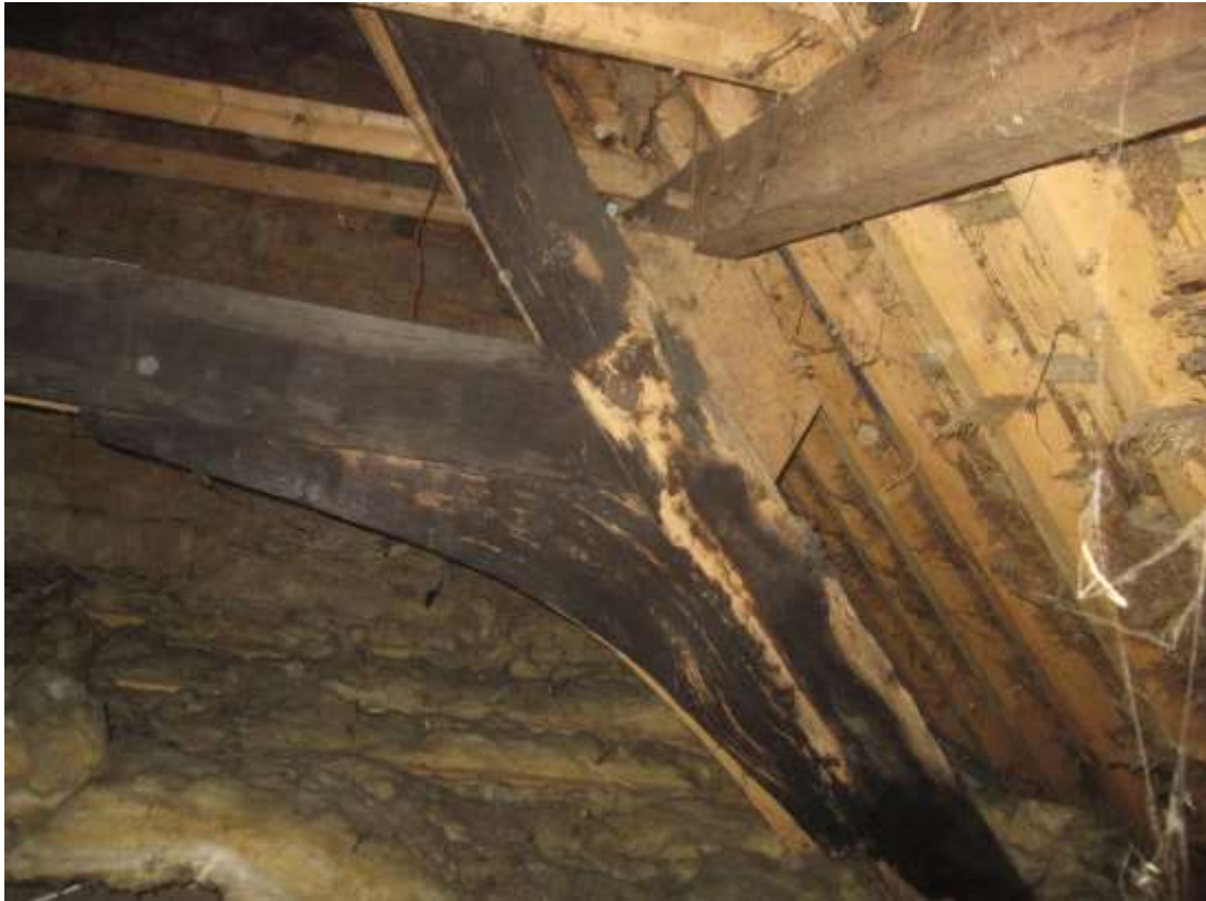
Truss T3 with arch-brace
