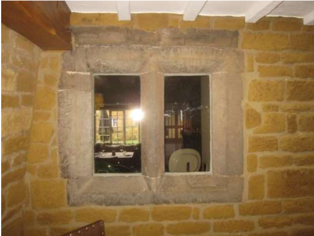
The east (external) face of the mullioned window of the north room (parlour)
