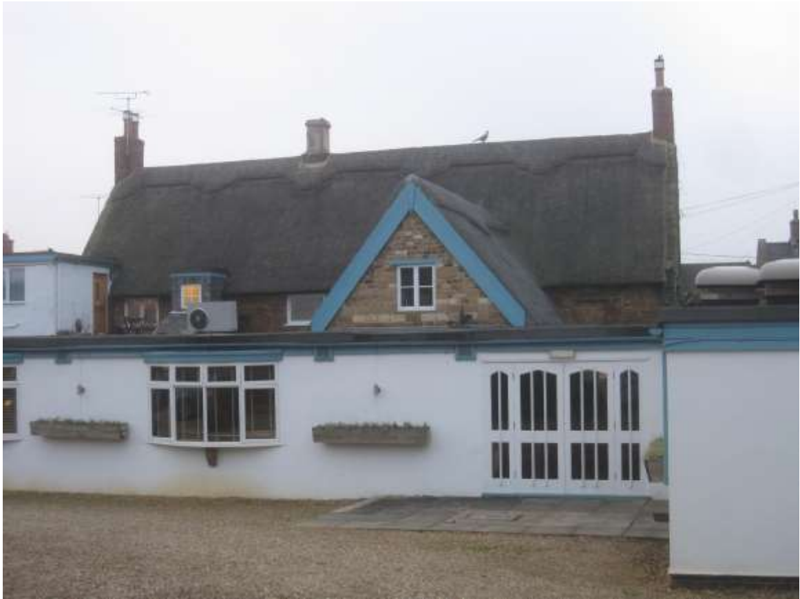
View of rear
