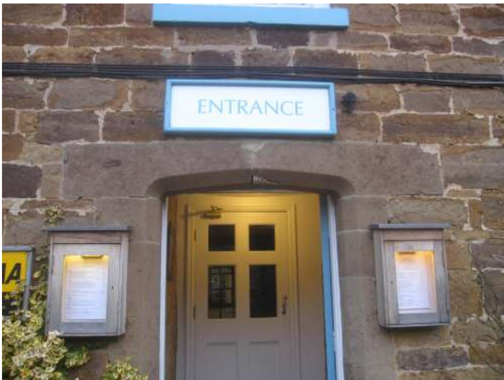
The front doorway
