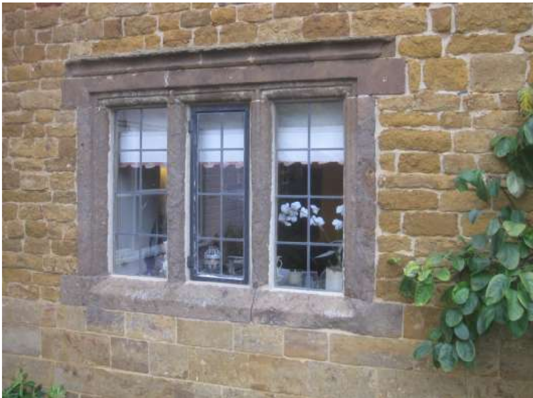
Stone mullioned window to east front
