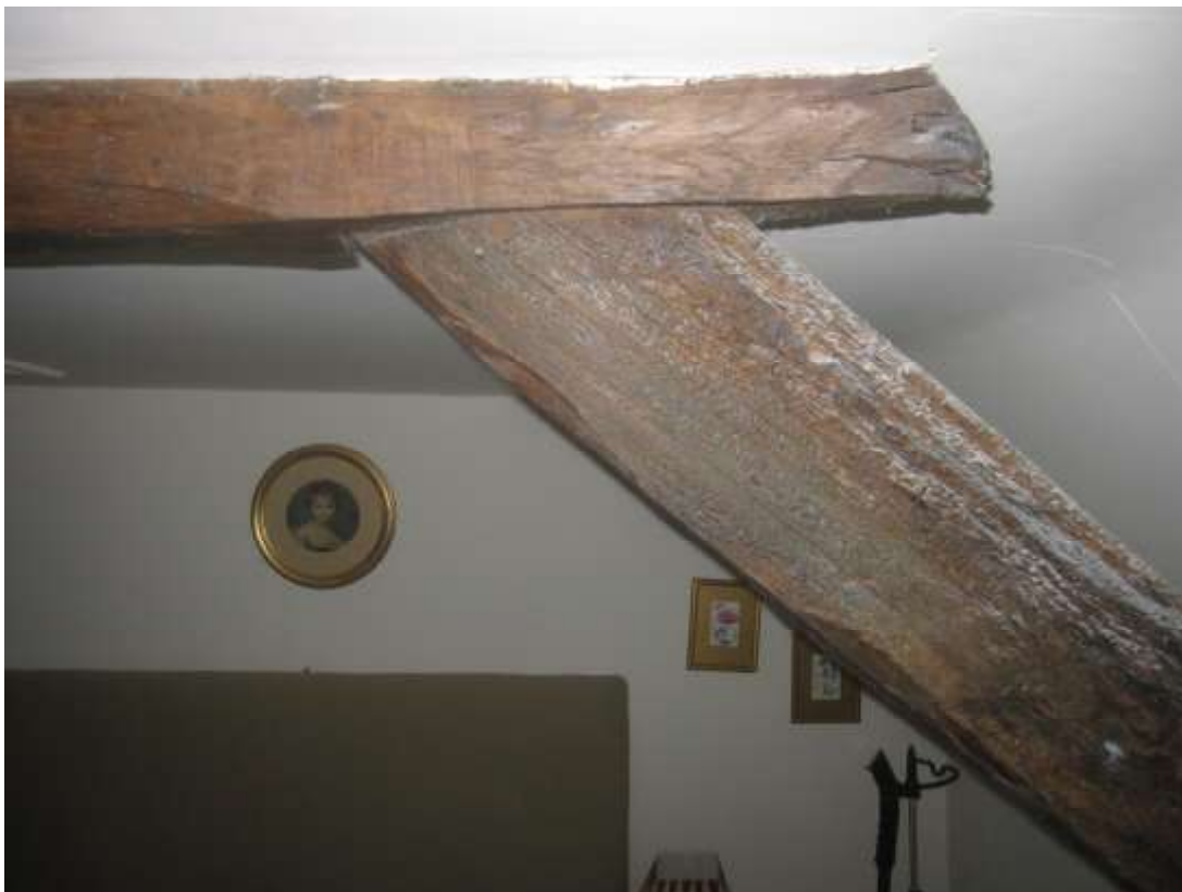
Lap joint to collar/principal rafter of truss T1
