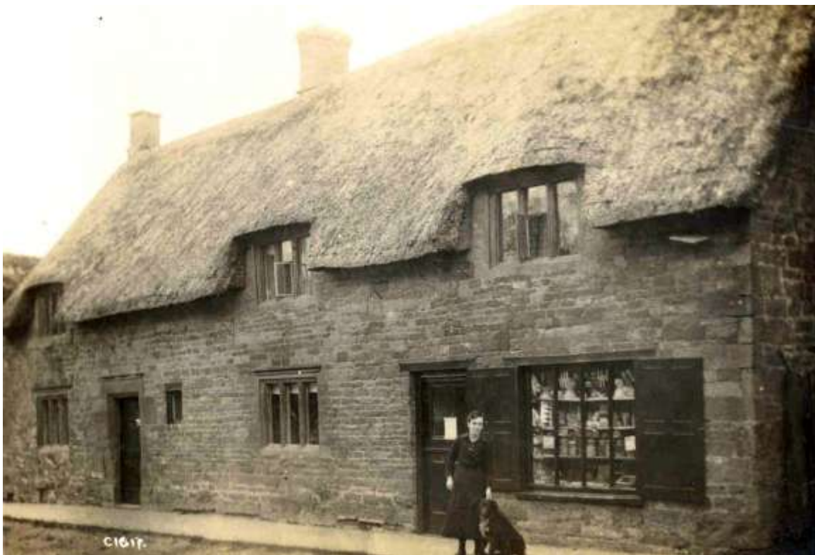
The former Post Office to the north end
