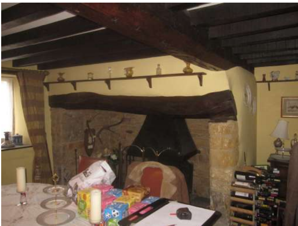
Inglenook fireplace in the south room
