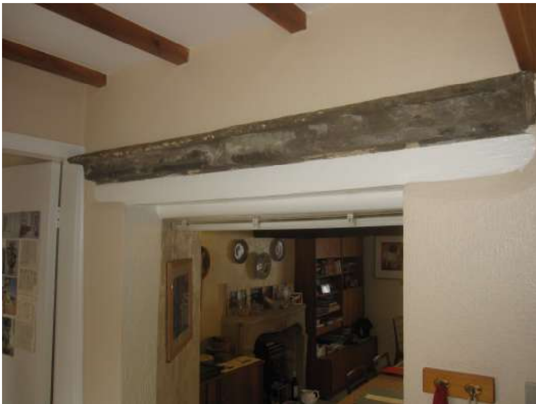
17 th century moulded cornice over former window in west wall of north room
