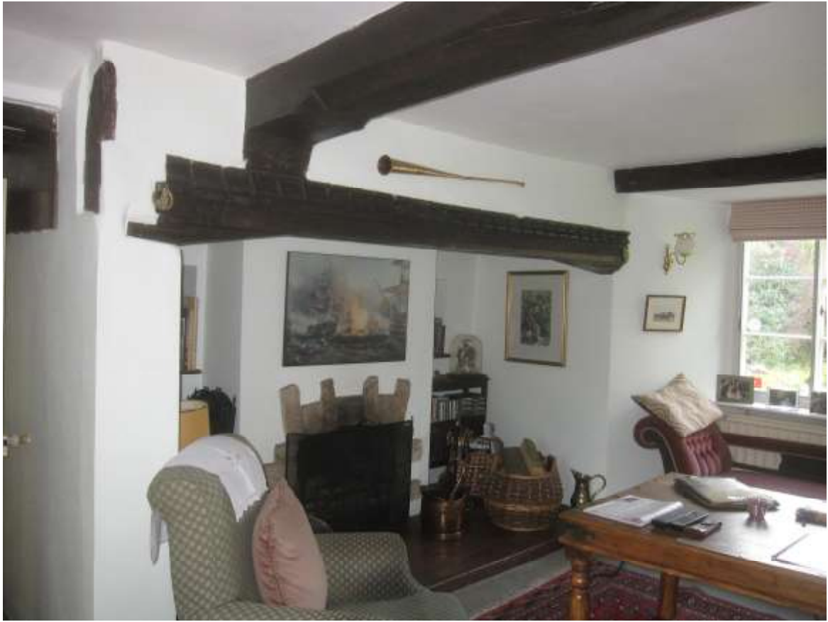
The inglenook fireplace with re-used embattled beam
