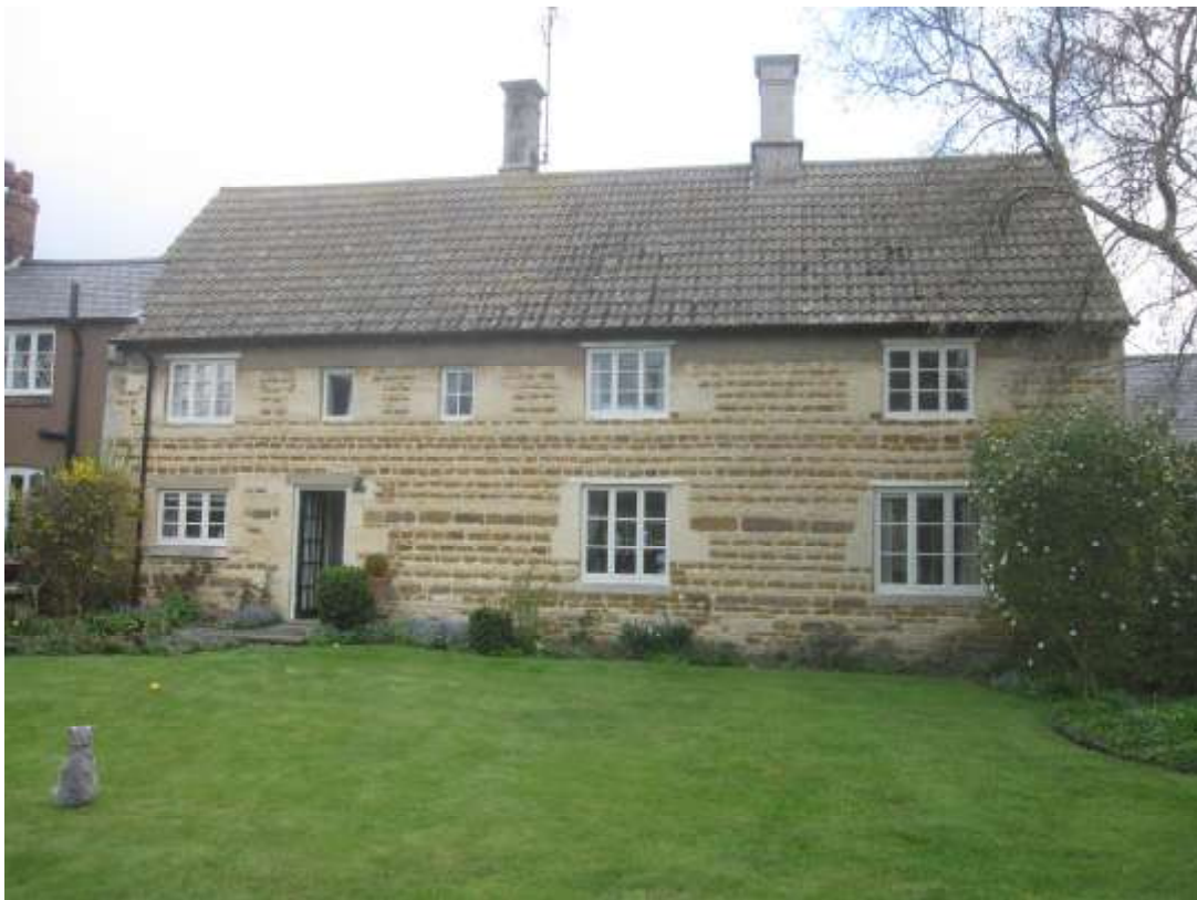
View of the rear from the south
