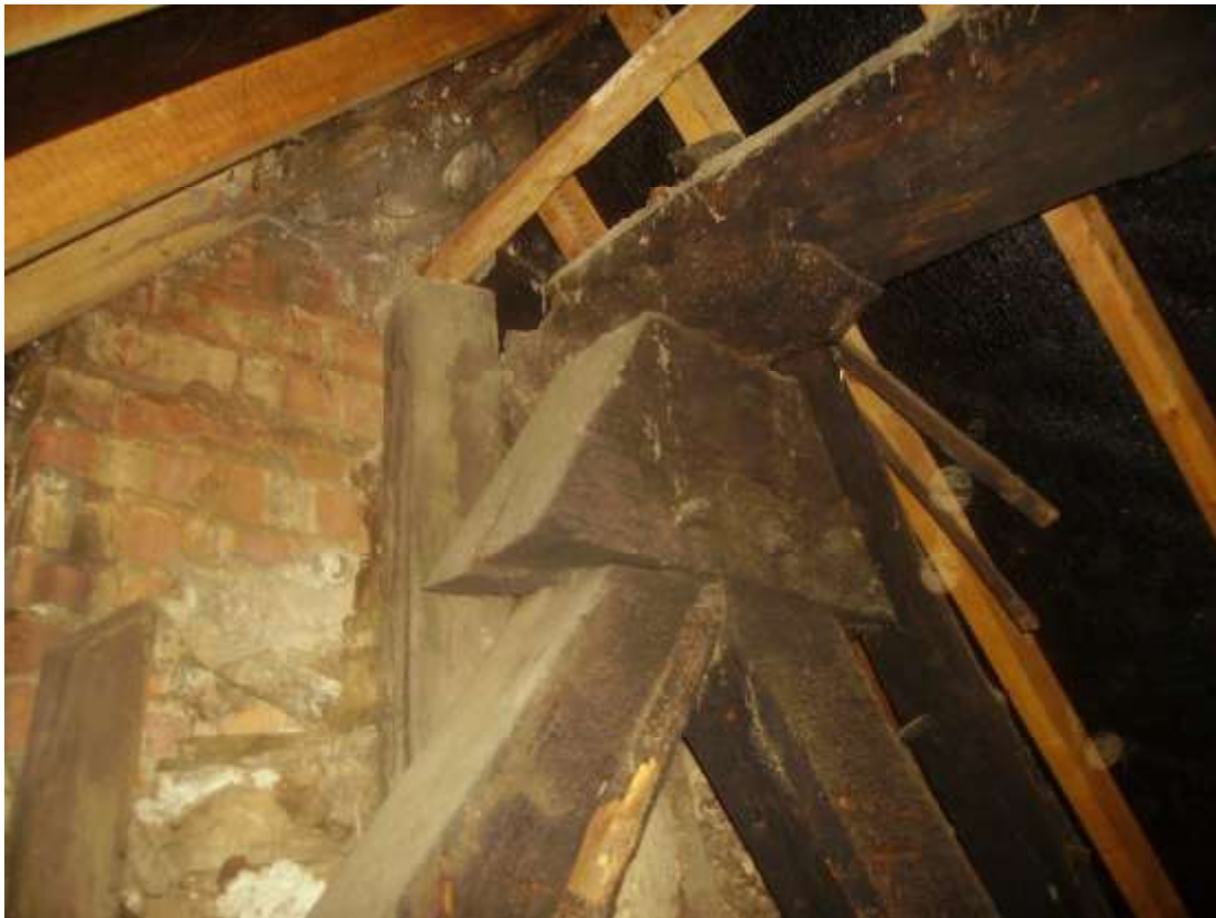
The apex of the cruck truss, with smoke-blackening
