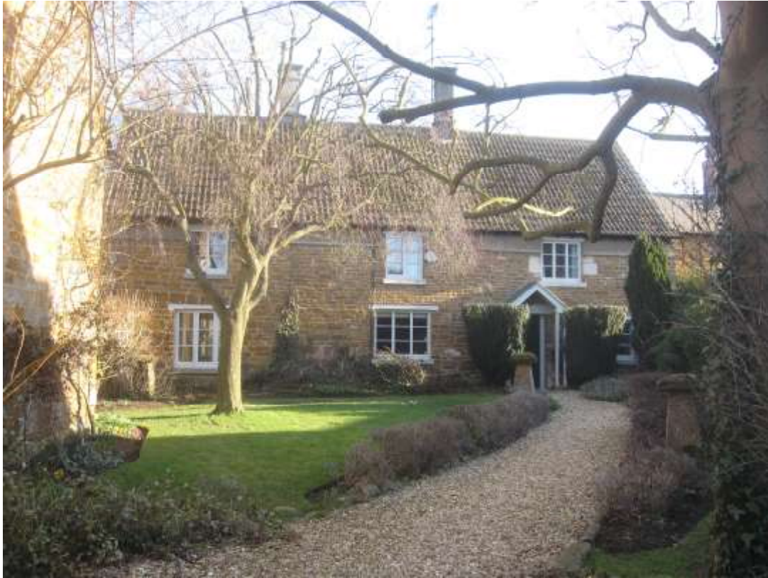
View of the north front
