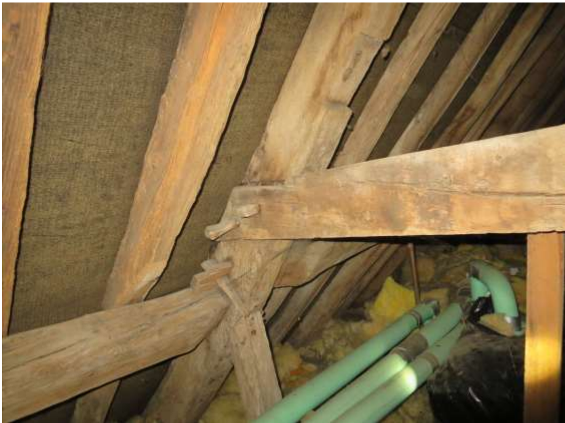
Detail of truss T3, south side
