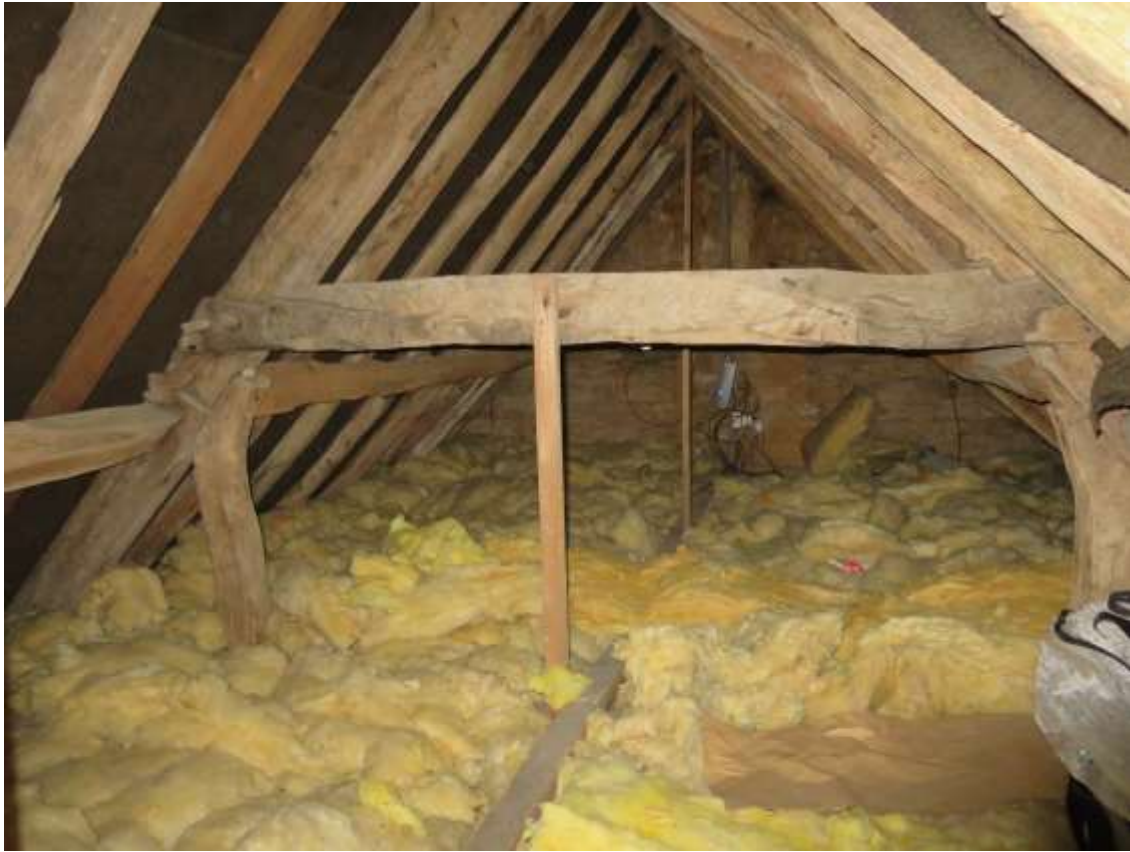
Truss T1 north side, with re-used curved struts
